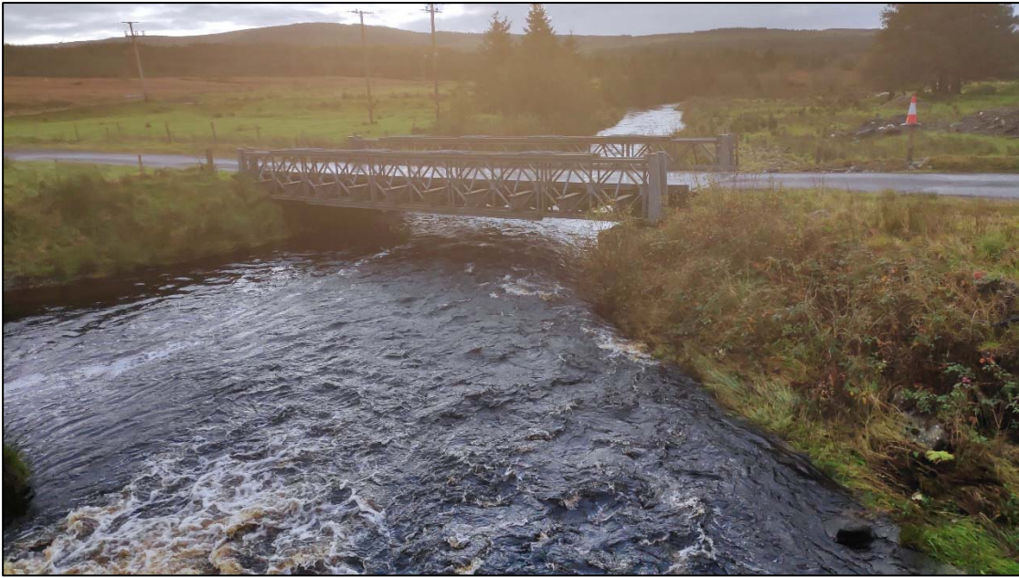
Plate 71: Bridge along which proposed haul route is located looking South. Road widening to take place to E and W of bridge along road.
