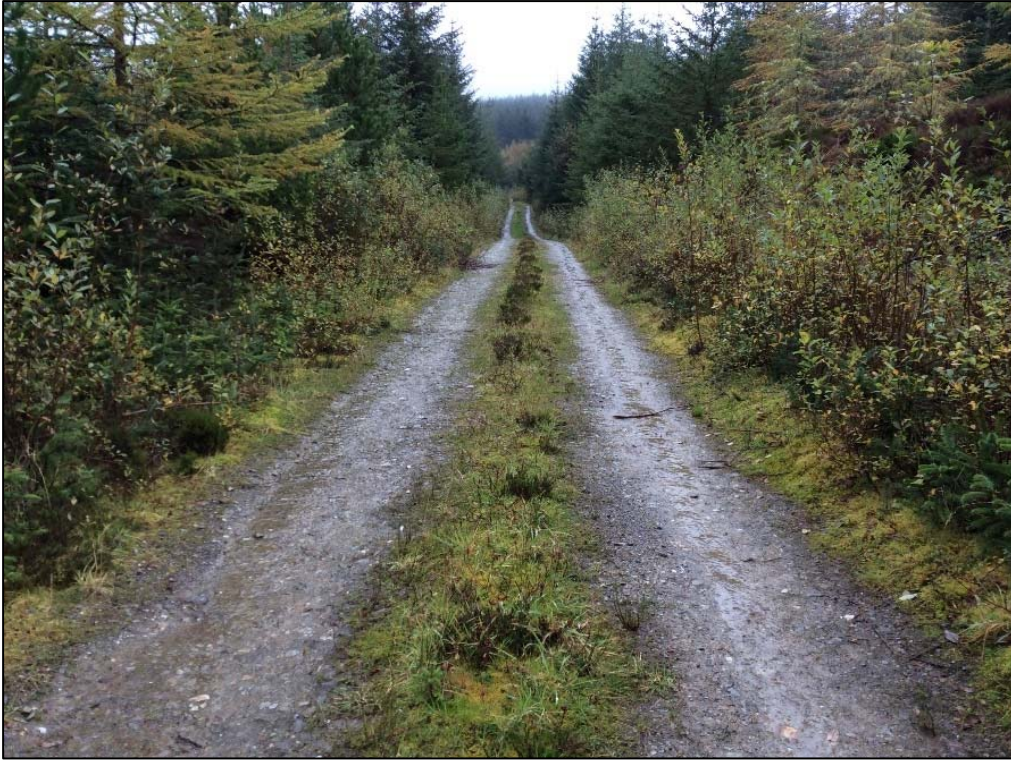
Plate 20: Existing forest road to the south of T8 turbine looking East.
