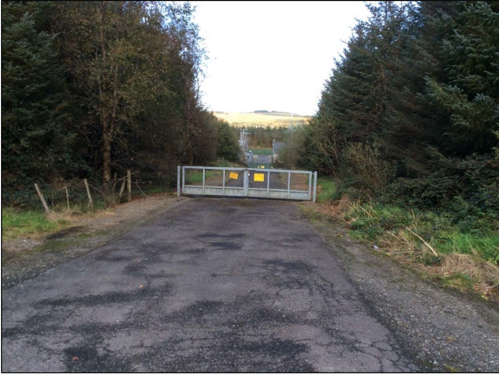
Plate 59: Trillick substation looking N.
