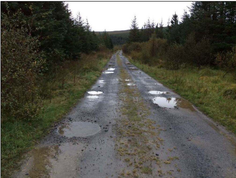
Plate 35: Existing road to the south west of compound looking south-east.
