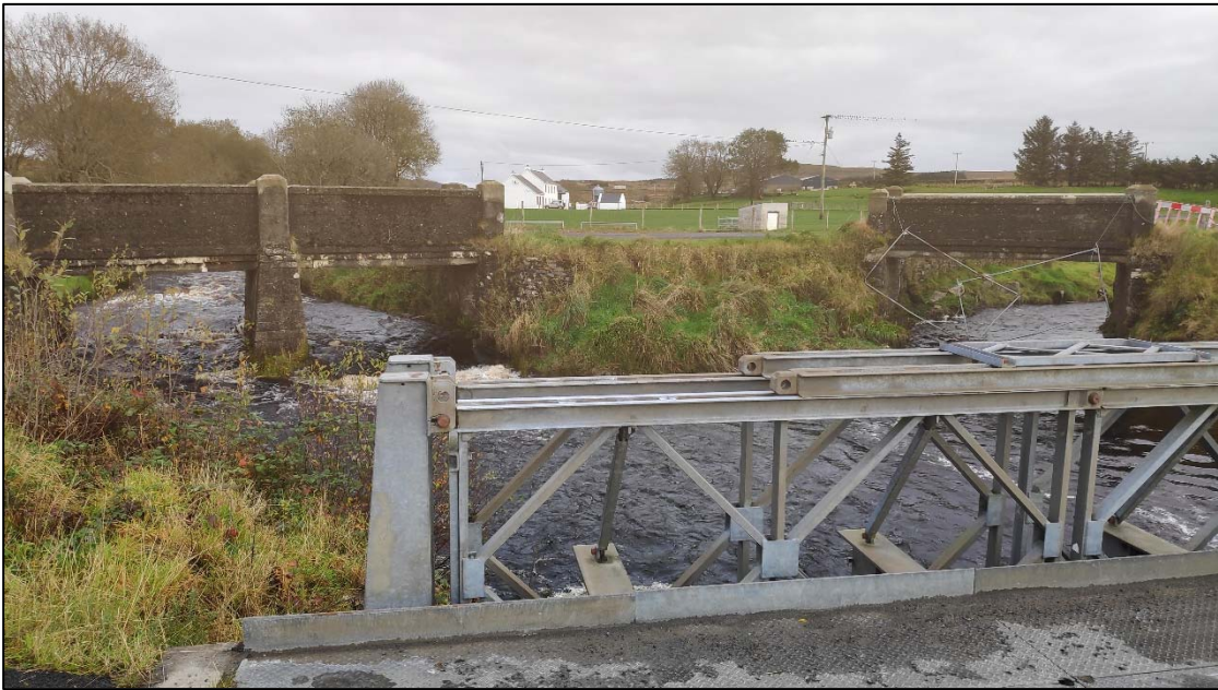
Plate 72: Wider metal bridge looking north at two smaller stone / concrete bridges.
