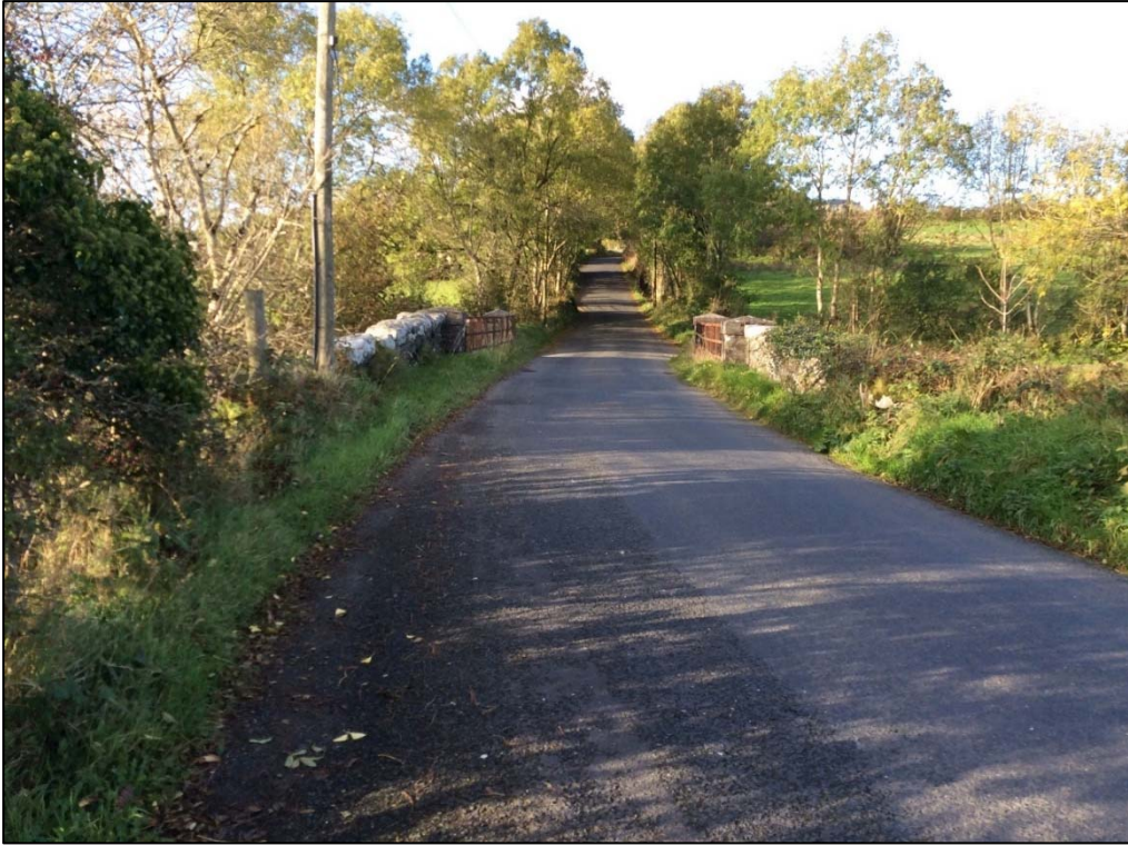
Plate 51: Same road bridge looking N (Tullydush Bridge).
